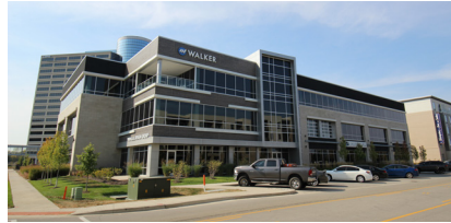
The Walker Building / Source: CoStar
